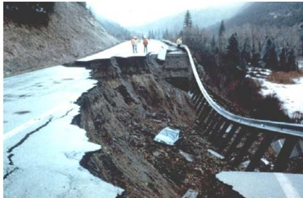
Slope failure near McClure Pass, Colorado (The National Landslide Hazards Program 2002)
